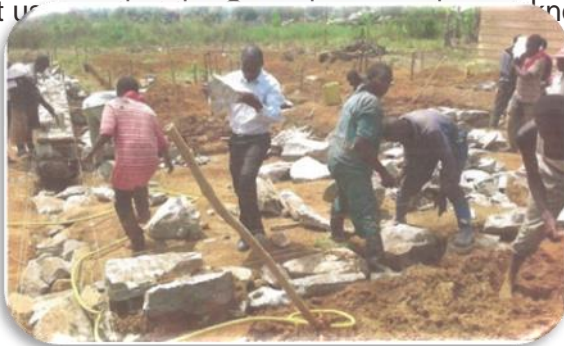
BREAKING GROUND AT THE NEW SCHOOL IN BENI
